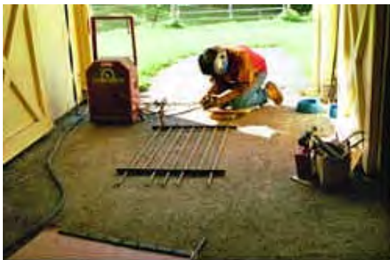
Jerry welds the cell bars to the horizontal pieces
