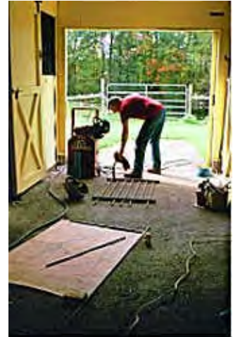
Jerry sets up his welder while Deb cuts the steel to size
