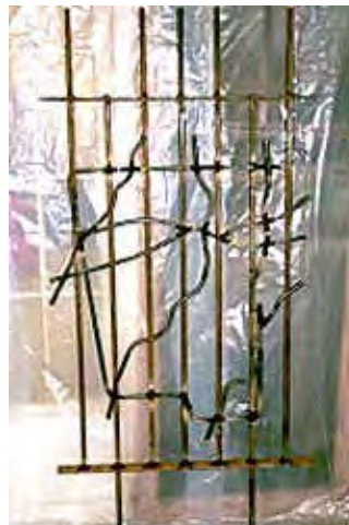
Jerry's finished welding job
